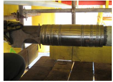
Secondary Marking Inspection
