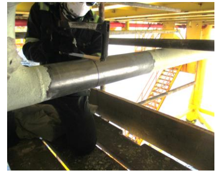
Cutting the pipe with hack saw
