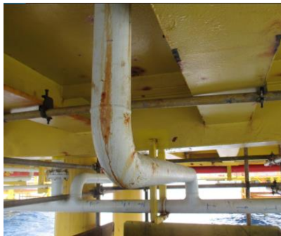
Identifying the pipe to be cut
