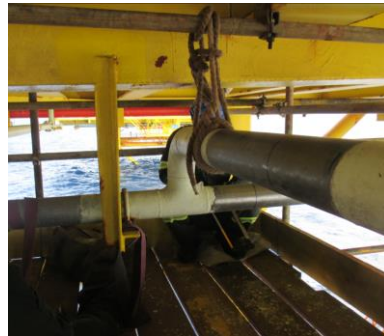
Surface Preparation to bare Metal
