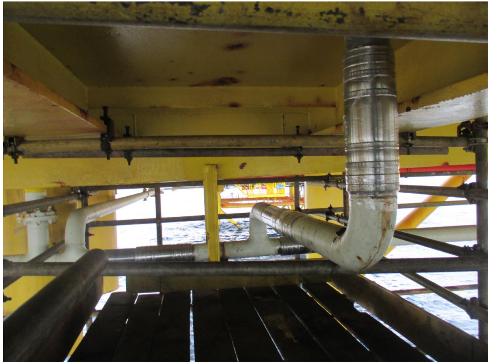
View of the Installed Pylok® Fitting
